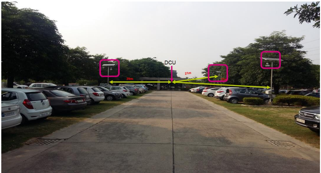
Fig ANNEX5.3: Implementation in the field, STMicroelectronics Parking at Greater Noida, INDIA
